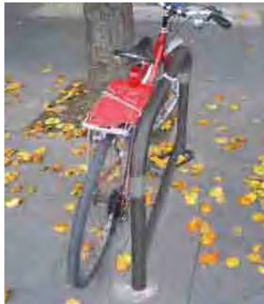
Figure 8.3 Sheffield stands are simple and effective. The design allows the bicycle frame and wheels to be easily locked to the stand. Note the tapping rail near ground level and the reflective bands on the uprights.
