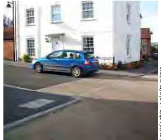
Figure 7.11 Quadrant kerbstones used instead of large radii at junctions reduce the dominance of the carriageway. This is reinforced by the placement and form of the adjacent buildings and the absence of road markings. However, note the lack of dropped kerbs and tactile paving.
