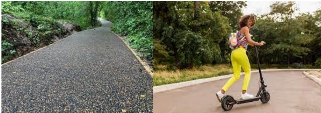
Suds Surface (left photo): such as Conipave or Flexipave are well drained and natural looking using stone and rubber.
