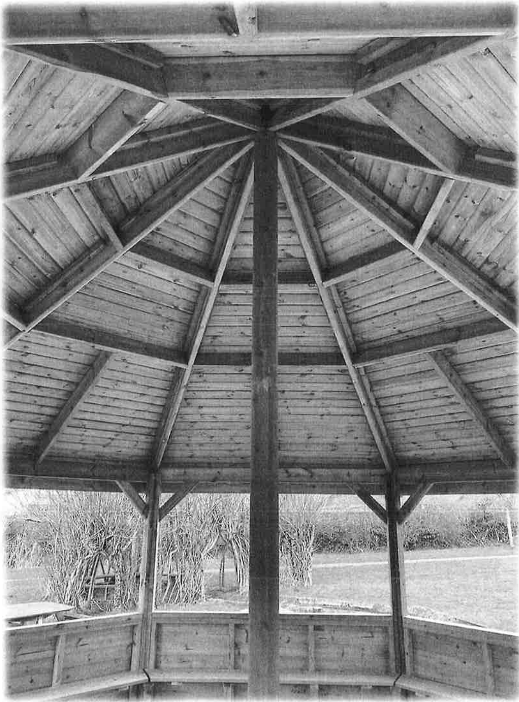
Ceiling in tanalised grade 4 pine log with central support post
